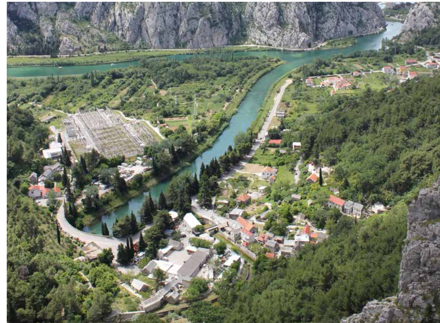
Zakučac hydro power plant on the river Cetina
